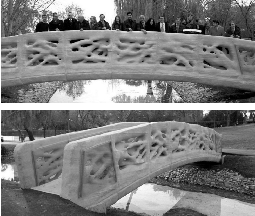
Fig. 8: In Spain, the First Pedestrian Bridge Printed in 3D in the World (3D BRIDGE) was Inaugurated 14th of December of 2016 in the Urban Park of Castilla-La Mancha in Alcobendas, Madrid
